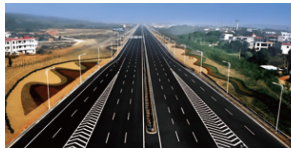
Ruili to Menglian Expressway Electromechanical Project
