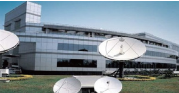
Shanghai Securities Waigaoqiao Earth Station
